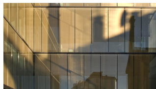
C Quadro, Executive Building, Udine, IT
